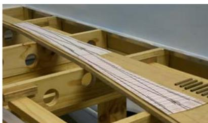
*This photo shows the photocopied paper templates attached to the 3mm MDF insert with sticky tape. I suppose you could glue the paper template in permanently but I felt this was unnecessary and I didn't want anything to change the rail height suddenly, even something as thin as a piece of paper. So I attached the template temporarily in place with*
